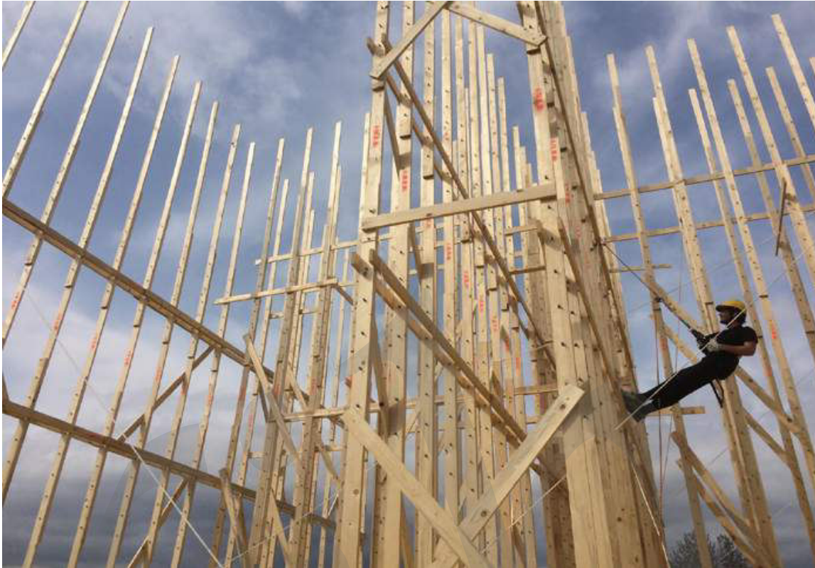
Fig. 1 Vectors. Construction site of House 1 (House 1, EPFL Campus, Lausanne, 2016)
