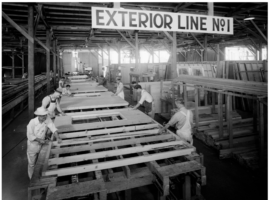
Assembly area, Workers assemble walls for houses in a warehouse of Kaiser Community Homes, Los Angeles, 1946. Photo: Dick Whittington Studios
