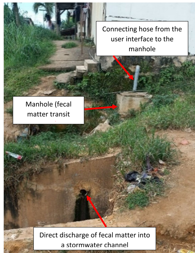
Fig. 2 Example of unhygienic/unsafe emptying: emptying of fecal sludge into open drains via illegal connection in study area
